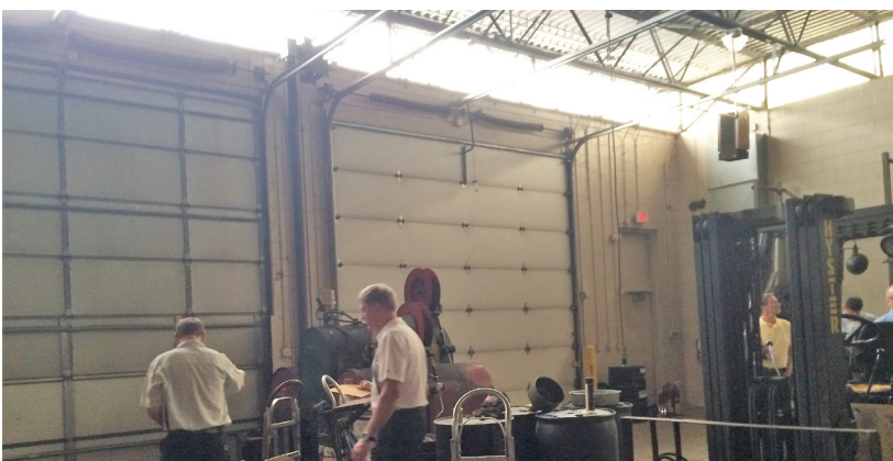
clerestory panels replaced, existing openings repurposed
