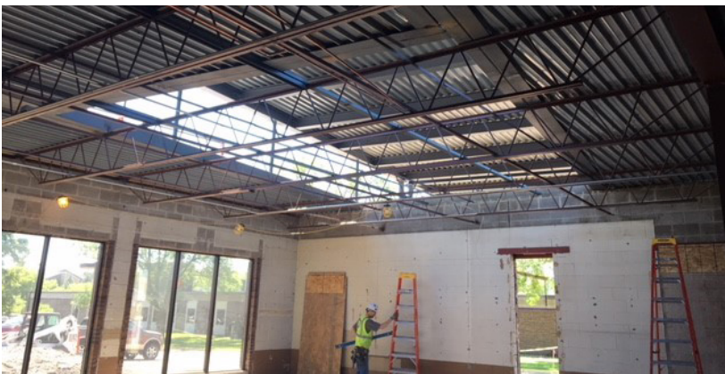
new elevated roof with clerestory panels and curtainwall entrance
